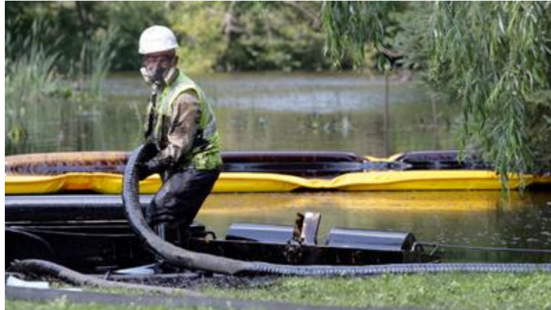
A worker from Enbridge skims oil off the surface of the Kalamazoo River after a pipeline ruptured in Marshall, Michigan. (July 27, 2010) - photo Andre J. Jackson/MCT
