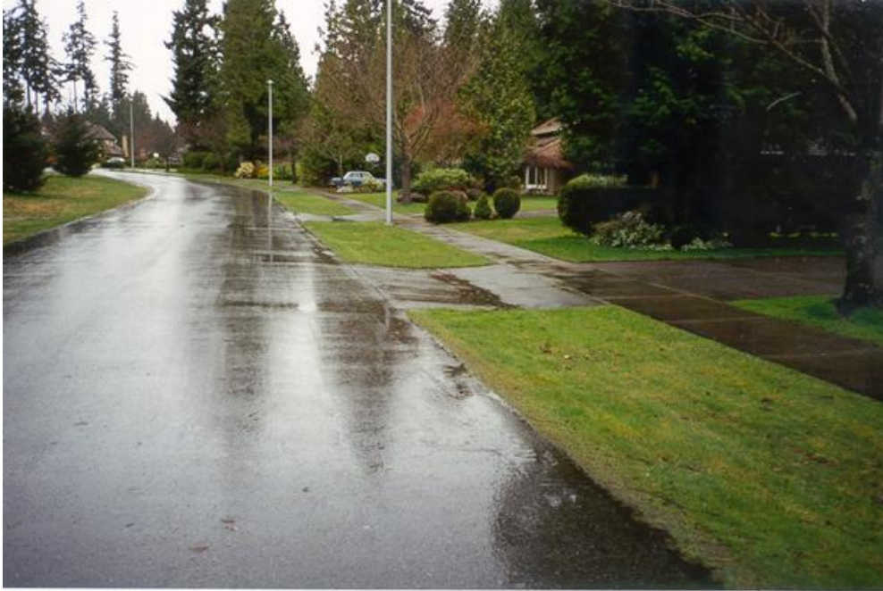
The salmon-friendly boulevards of Surrey's Amble Green. For a more detailed look at the project go here .
