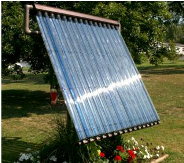
Solar hot water systems use a thermos-like setup to catch the energy of the sun. (Photo courtesy of Earth Energy Innovations.)
